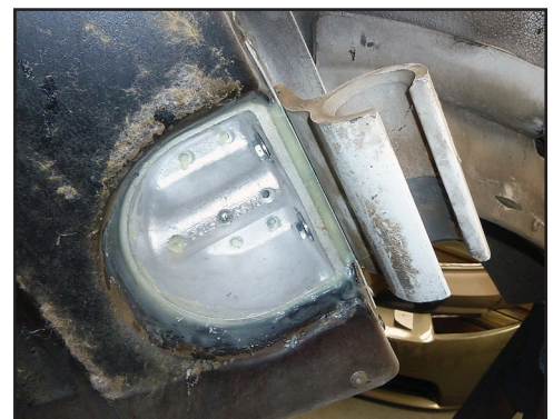
A job well done and ready for the road. Congratulations, you just saved a lot of time and money!
