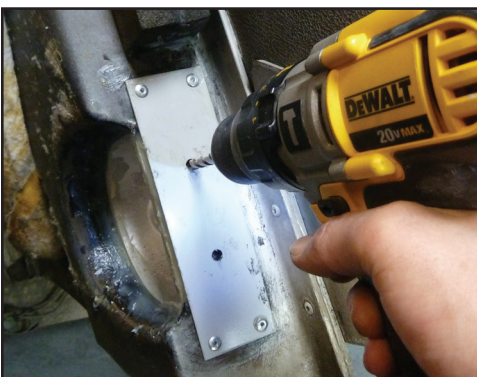
Re-drill the bolt holes with a 5/16" drill bit.
