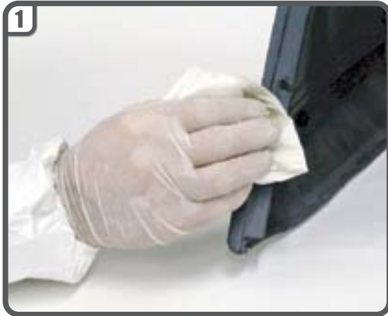
1 Use lint-free cloth to prepare surface with Water-based S2000 .
